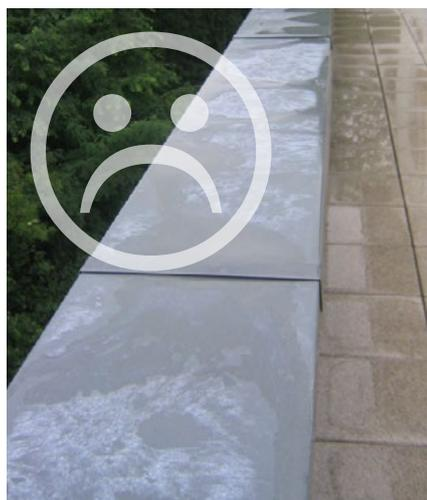
Zinc hydroxide formation due to insufficient slope
