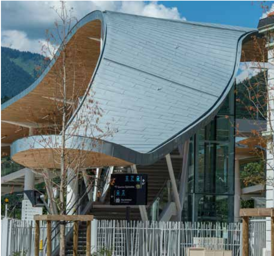
Passerelle, Cluses, France
