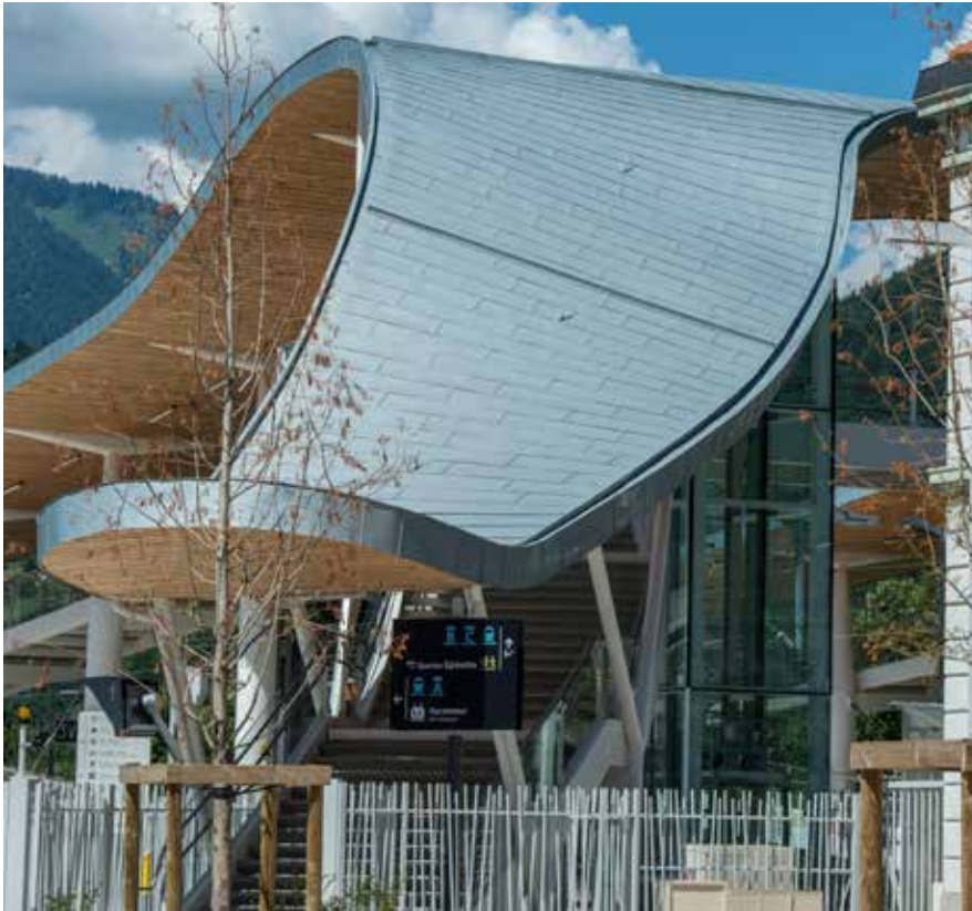
Passerelle, Cluses, France
